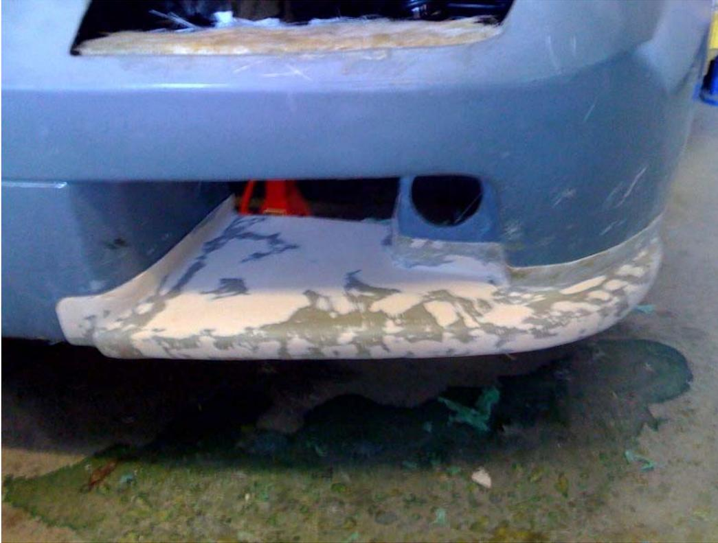
Surface is sanded to prepare for manufacture of the carbonfiber panel
