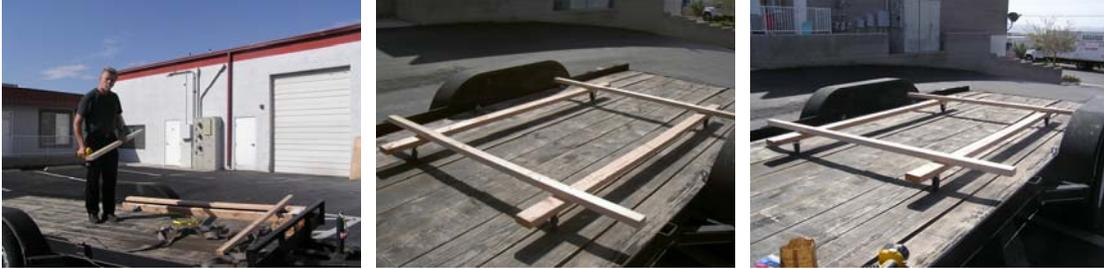
The body is lifted on the trailer and the short range body pallet is inserted under the body and secured in 4 corners with screws and fender washers.
