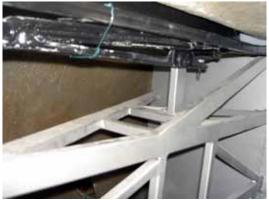
We used wire ties to keep the hinges in the compressed position, once they were mounted to the upper support with the metal screws.
