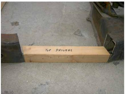
After the block is cut, try fitting it in the planned area that the square metal tube will be welded.
