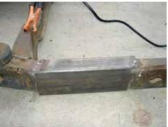
When alignment and spacing is proper, tack weld the extension tube.
